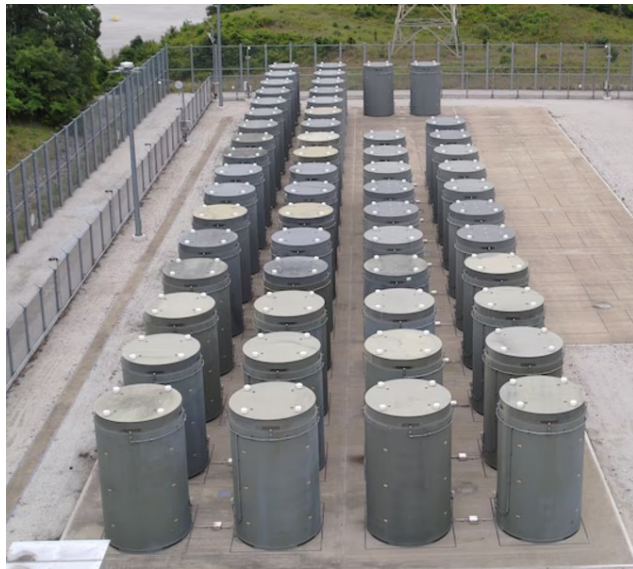
Casks storing spent fuel at the Donald C. Cook Nuclear Power Plant in Bridgman, MI. Image credit: Appalachian Power Company
