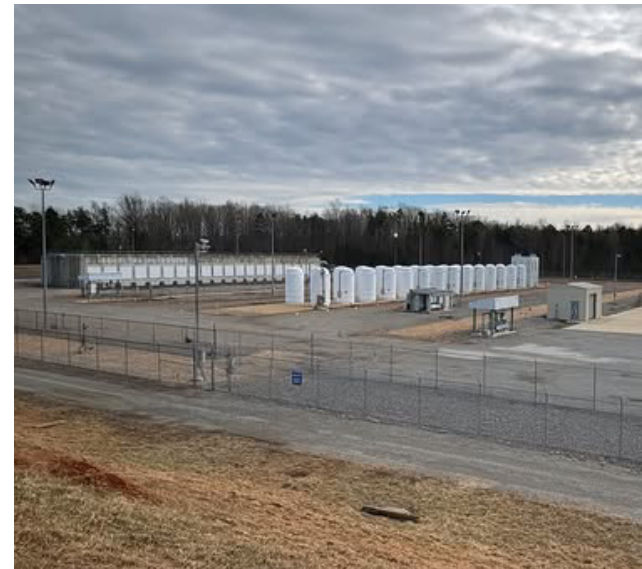
Casks storing spent fuel at the Dominion Energy North Anna Power Station in Mineral, VA. Image credit: U.S. Department of Energy
